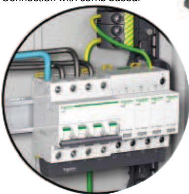
Surge arrester iPRD 4P + iC60N 4P
